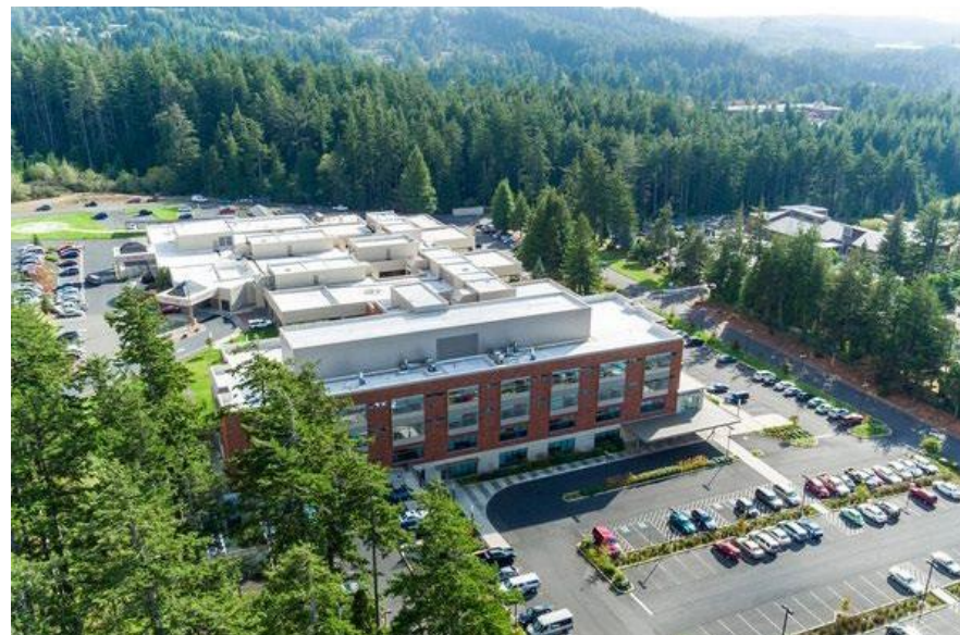
Figure 1. Bay Area Hospital, via Bay Area Hospital Website
