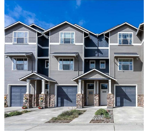
Figure 21. Townhomes, via Apartments.com
